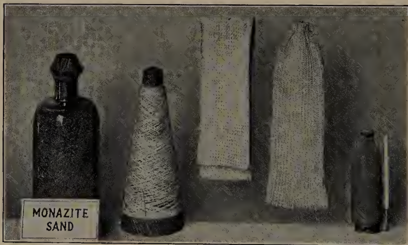
FIG. 120. Materials used in making gas mantles, and stages in the process of manufacture
